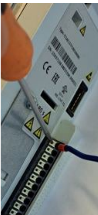
Push in connector with a screwdriver
