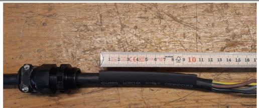
4 Install cable and shrinking tube with cable gland.
