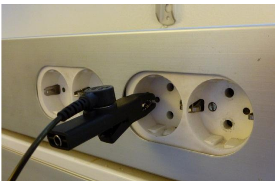
Picture 2: ESD mat connected to ground.
